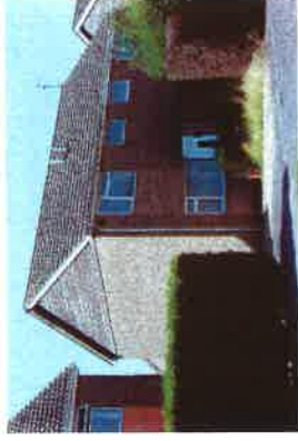
Semi-detached dwelling built in light buff brick with reconstituted stone panel and timber panelling to gable.
