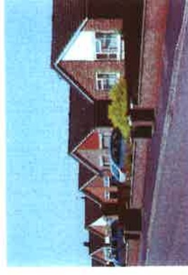
Mix of light buff and light brown brick with reconstituted stone, timber and PVCu panels as a contrasting material.
