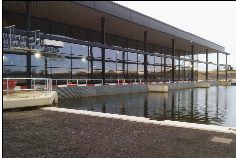
Photograph 5: New St Germans Pumping Station opened April 2010
