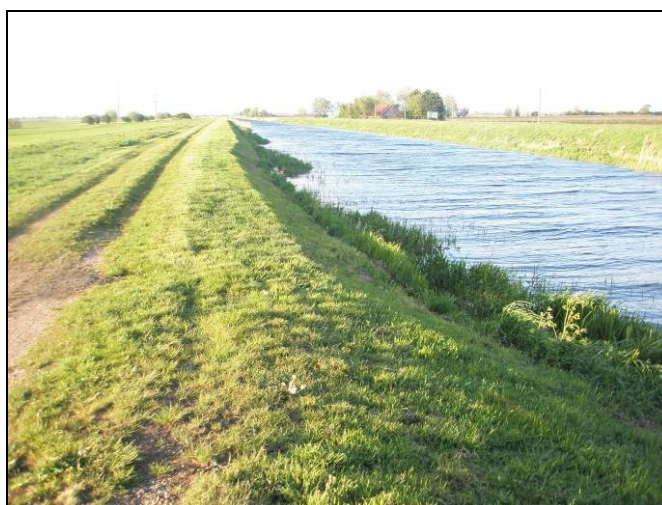
Photograph 4: Sixteen Foot Drain looking downstream from Boot's Bridge
