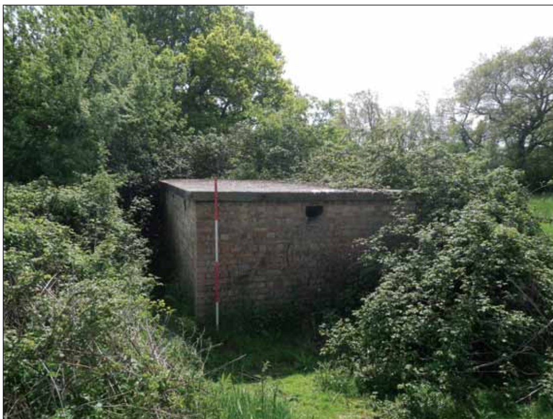
Plate 1: Home Guard Store in Field 1, facing south
