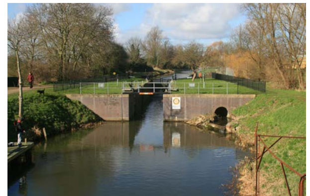
Ashline Lock Photo © Cllr Bob Wickes
