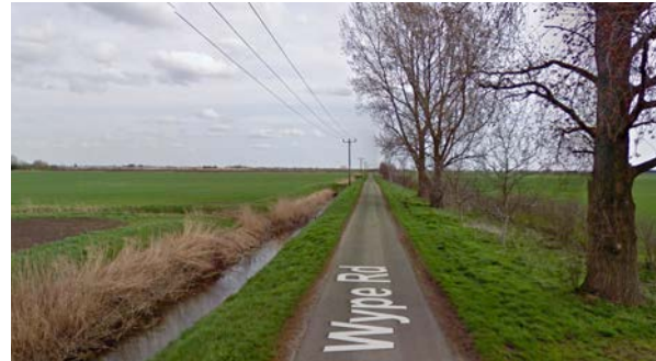
Example of local road between settlements: Wype Road
