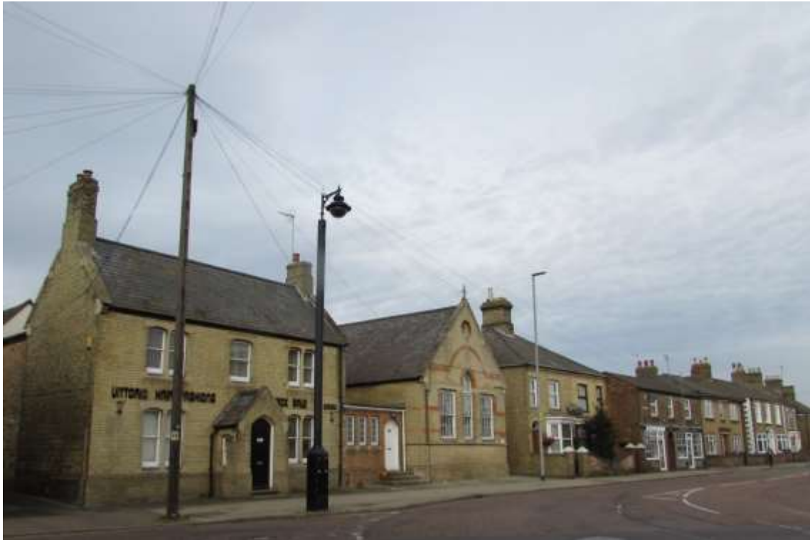
The 19 th Century former school building now a commercial premises and flats has a noticeable presence in the Broad Street scene
