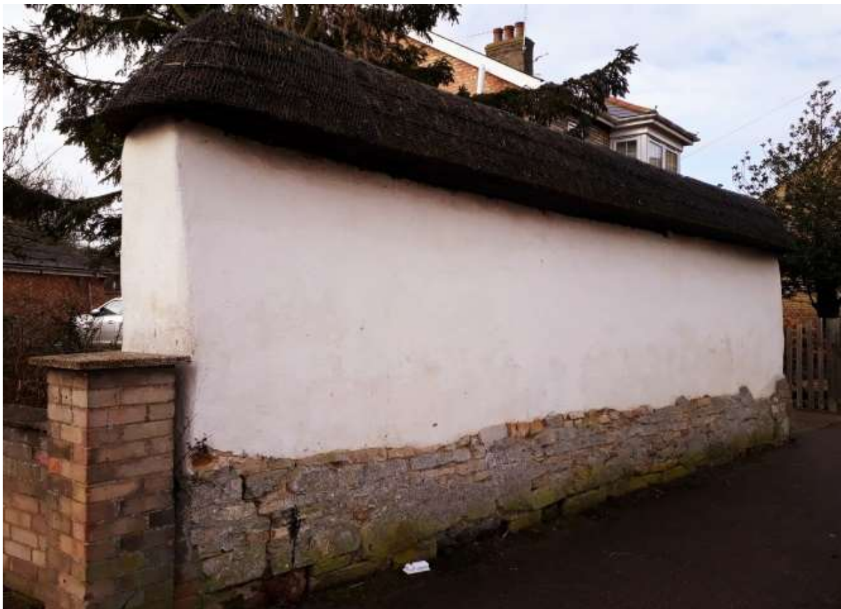
Mud walls are an intrinsic feature of Whittlesey's character. The wall on Delph Street is a well kept feature of the street scene.
