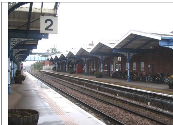
Station platforms looking east
