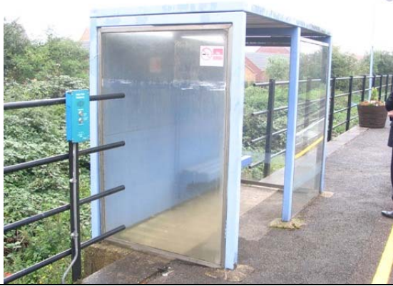
Down platform waiting shelter and seat.
