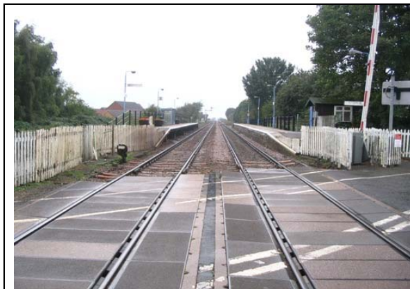
Overall view of station, looking northwards from Station Road
