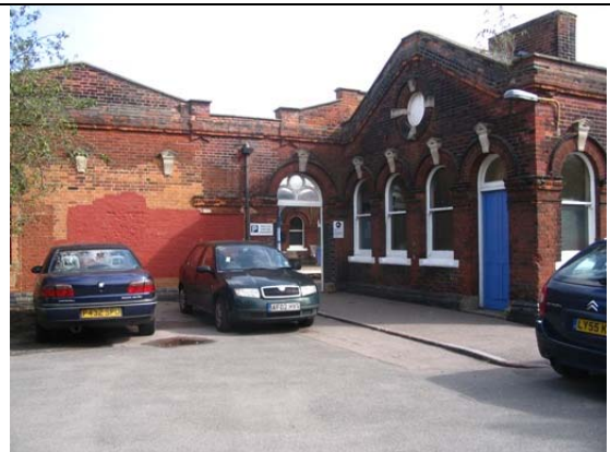
Out of hours exit from down platform
