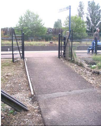
Ramped access to the up platform
