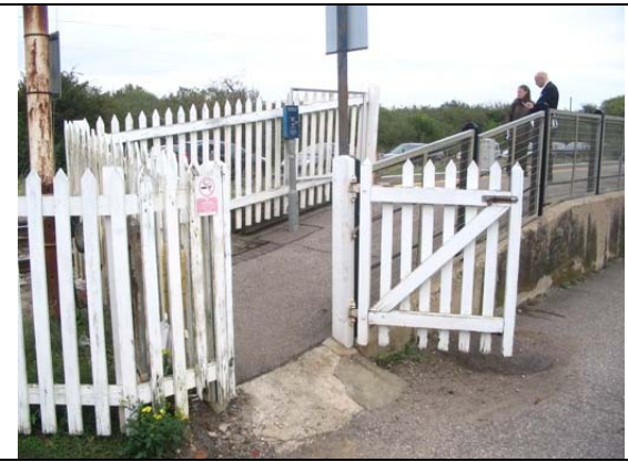
Down platform access gate and ramp.
