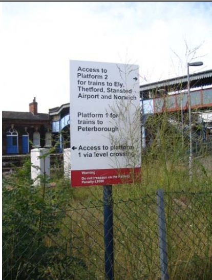
Access signage, up side
