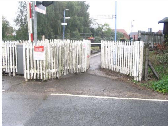
Access gate to up platform.
