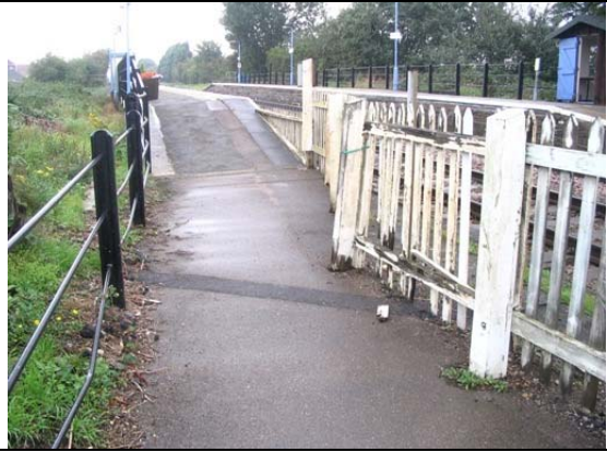
Down platform access ramp.
