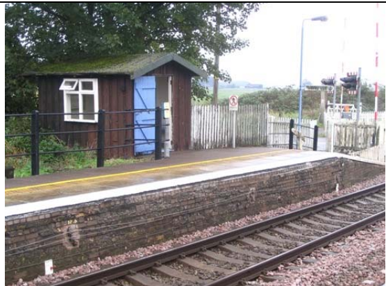
Up platform shelter.
