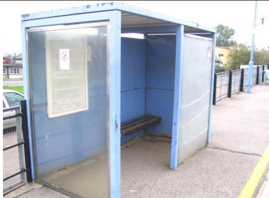
Down platform shelter.
