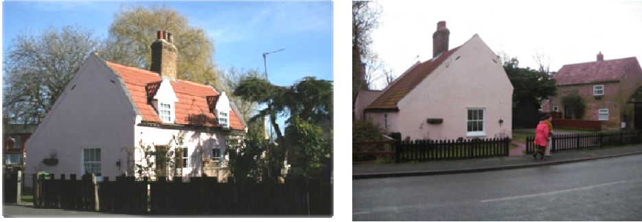
(LEFT) No.10 New Street, a Building of Local Interest (probably 18 th C) constitutes an interesting survival. No.12 (on the right) shows the remnants of the former farmhouse's rural setting with its open courtyard.
