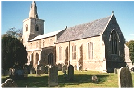
St Mary's Church south elevation
