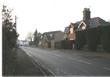
Westerly view along the southern side of Benwick Road, showing No's.1-3 in the foreground.
