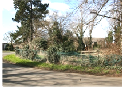
The deteriorating Church Lane Paddock boundary.
