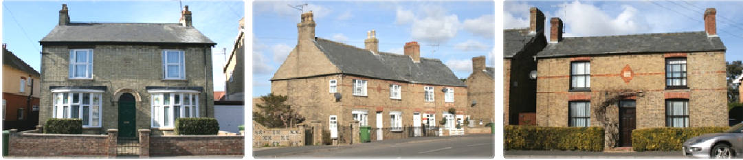
The use of a closely matched gault bricks and uniform Welsh slate in the construction of Nos.25-53 New Street enhances the group value of these buildings and serves to highlight their quality.
