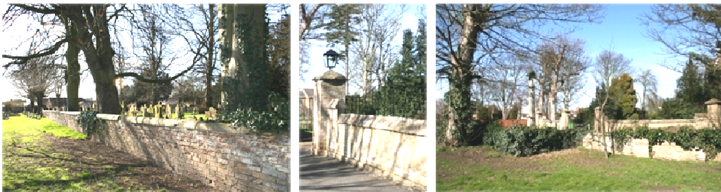
Historic boundary walls and dense tree canopies are extremely important components of the street scene in Church Lane.
