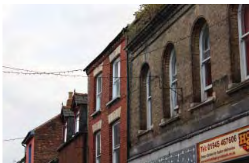
Windows at first floor level
