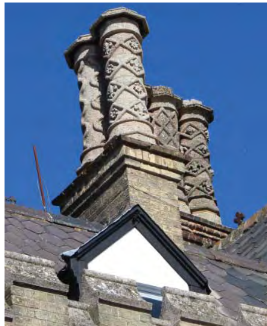
Elaborate chimney stacks on Nos.23-24
