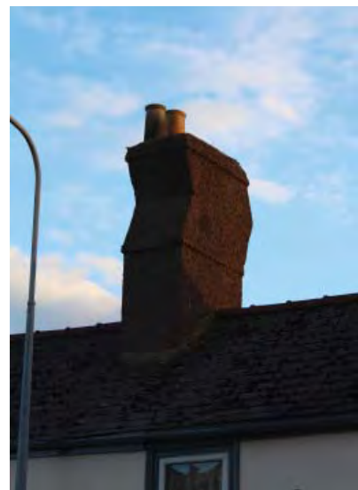
Chimney at Numbers 8-10 Blackfriars Road
