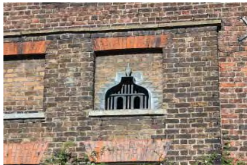
The Oggee Dovecote at No.11.
