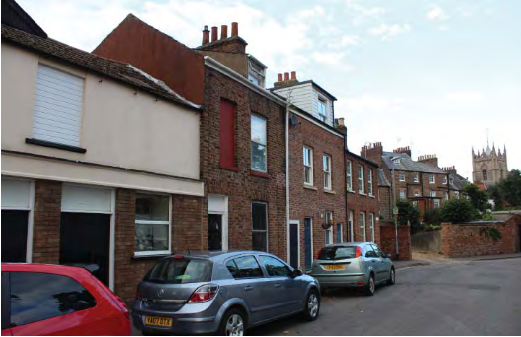
Buildings along Love Lane has suffered from a number of inappropriate alterations which detract from the historic character of the buildings
