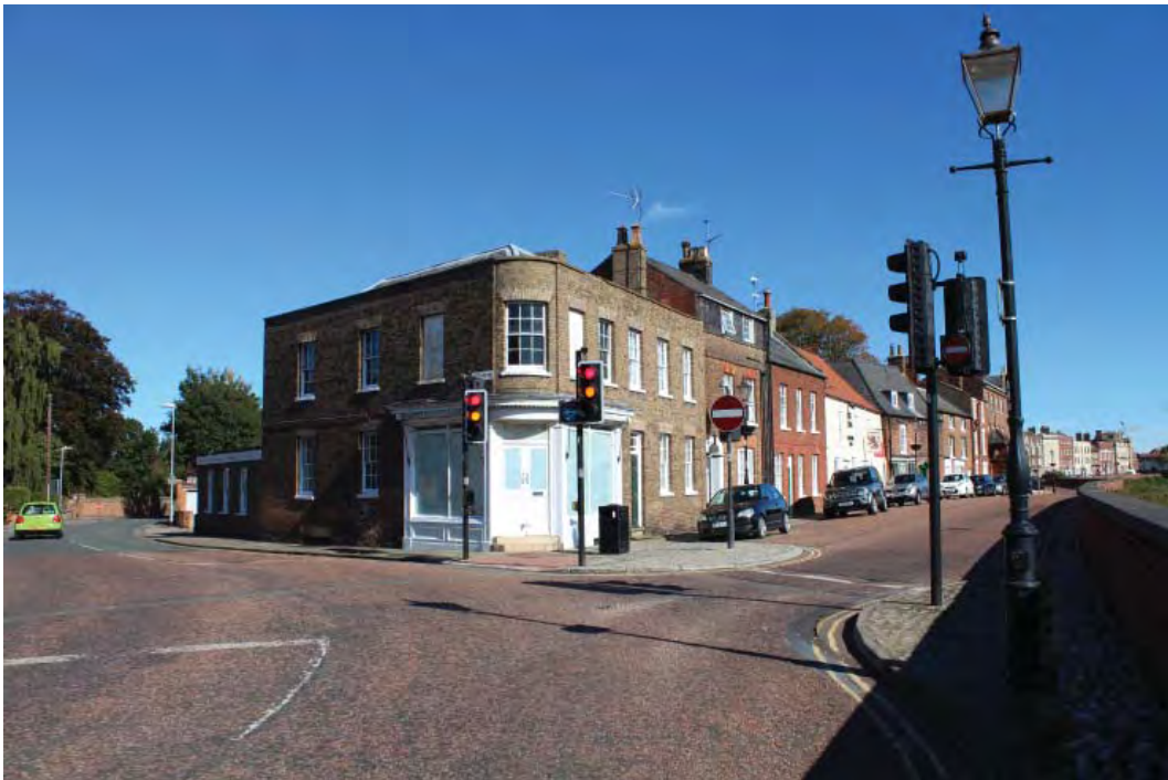
Street furniture and signage at the junction between North Brink and Chapel Road
