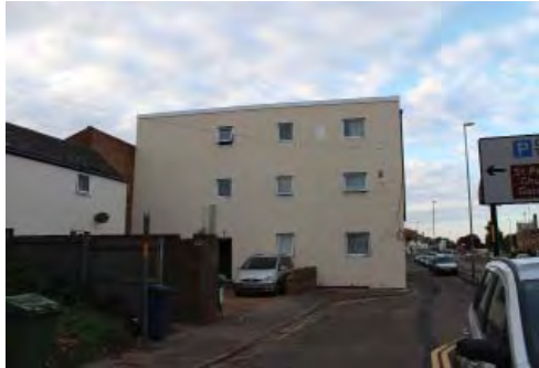
View looking north along Churchill Road. This building, clad in external insulation, does not contribute positively to the area
