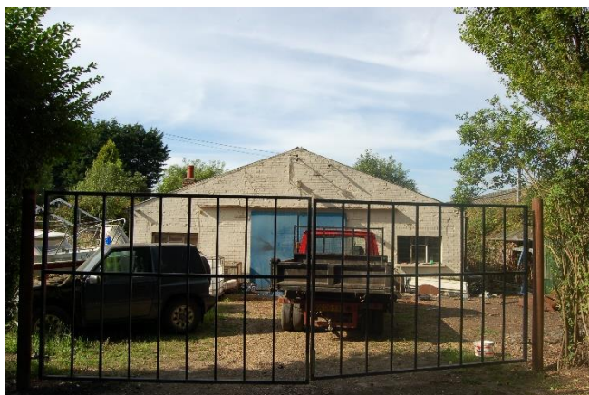
Photograph 15 Southern elevation of Building 4 looking north
