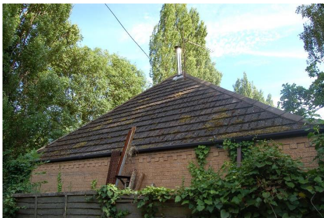
Photograph 13 Northern elevation of Building 1 looking south
