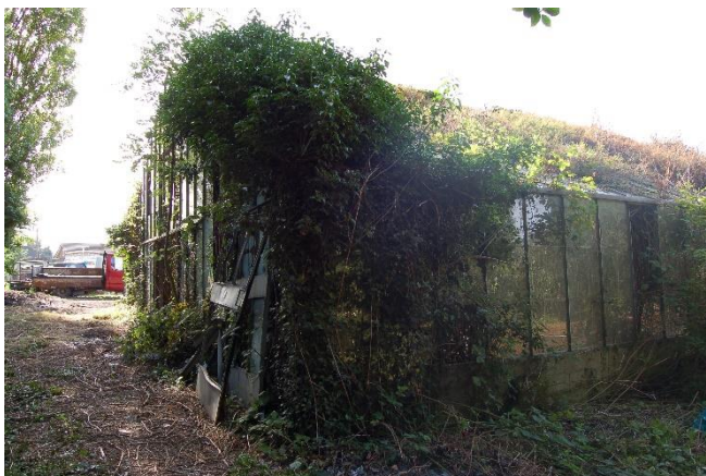
Photograph 16 Building 5 looking west
