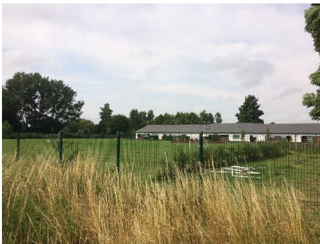
Photograph 17 Building 15 looking west
