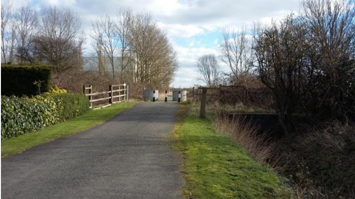
Figure 2.3: Disused Level Crossing
