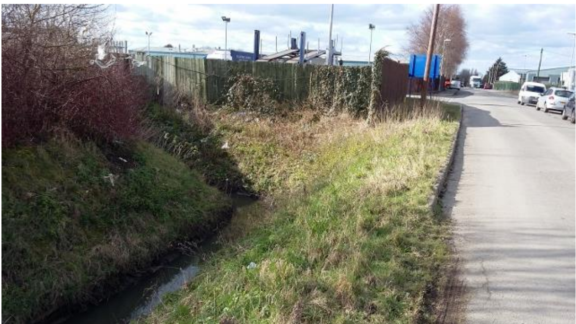
Figure 2.27: Drainage Ditch on New Bridge Lane
