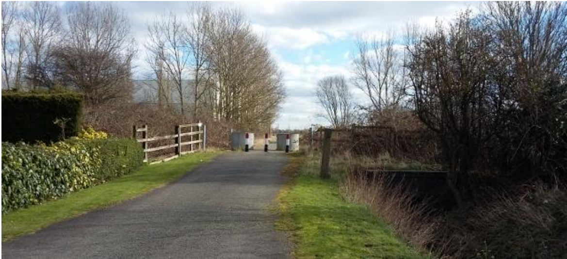
Figure 2.28: New Bridge Lane where it crosses the Railway Tracks
