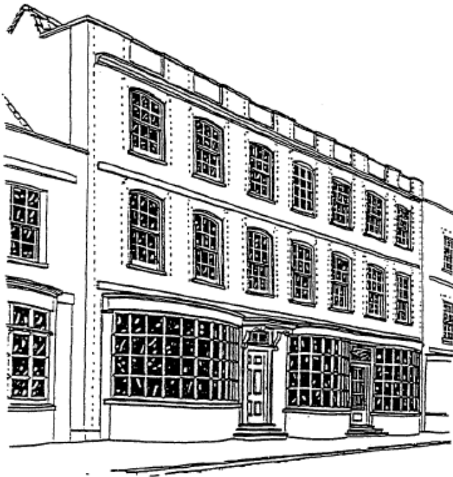
The same building from a photograph of 1856
